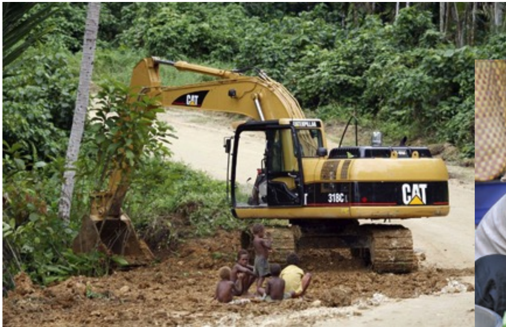
Building a road between Auki and Malu'u, Solomon Islands (credit: DFAT).
